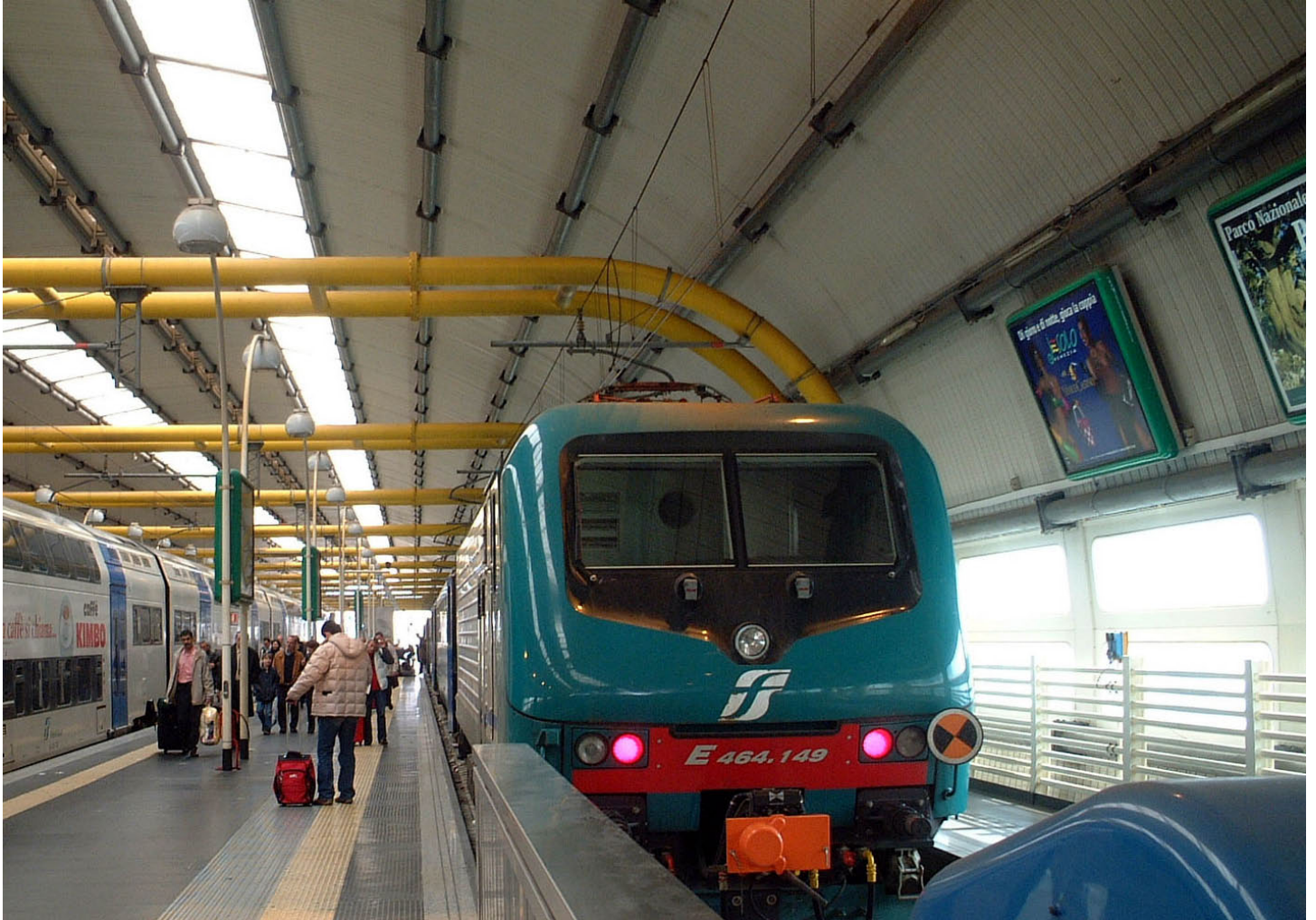
Railway Station at Fiumicino Airport - outside Rome
